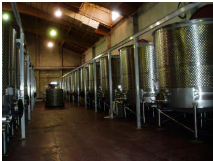
Left top: new plantings, Buena Vista House for guests in background; Right top, view of new plantings looking southeast toward San Pablo Bay; Middle: Old vine; Bottom: fermentation tank room.
